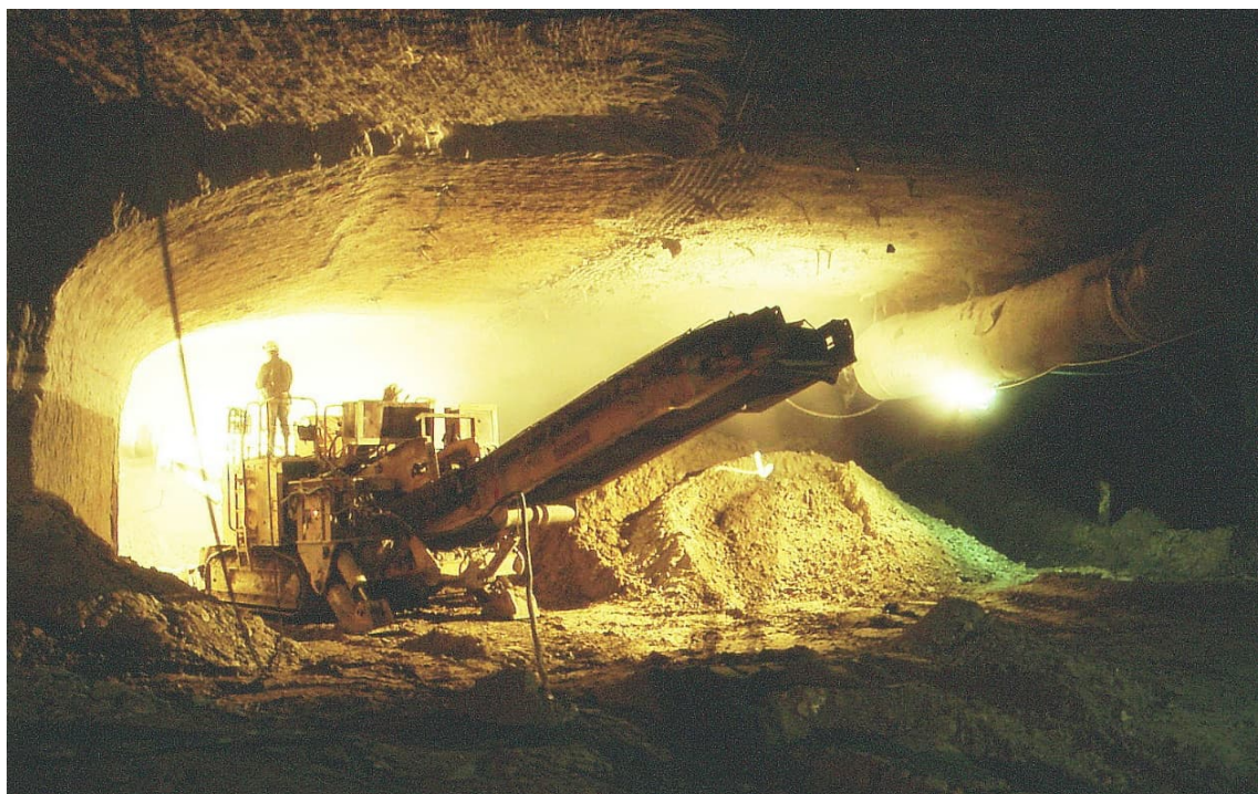
Figure 3. Excavating the crown of the cavern using Mitsui roadheader
