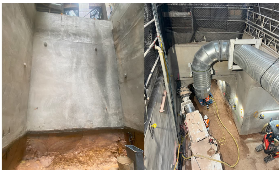
Figure 18: Photograph of the completed tunnel portal before tunnel breakthrough (left) and after tunnel breakthrough (right)
