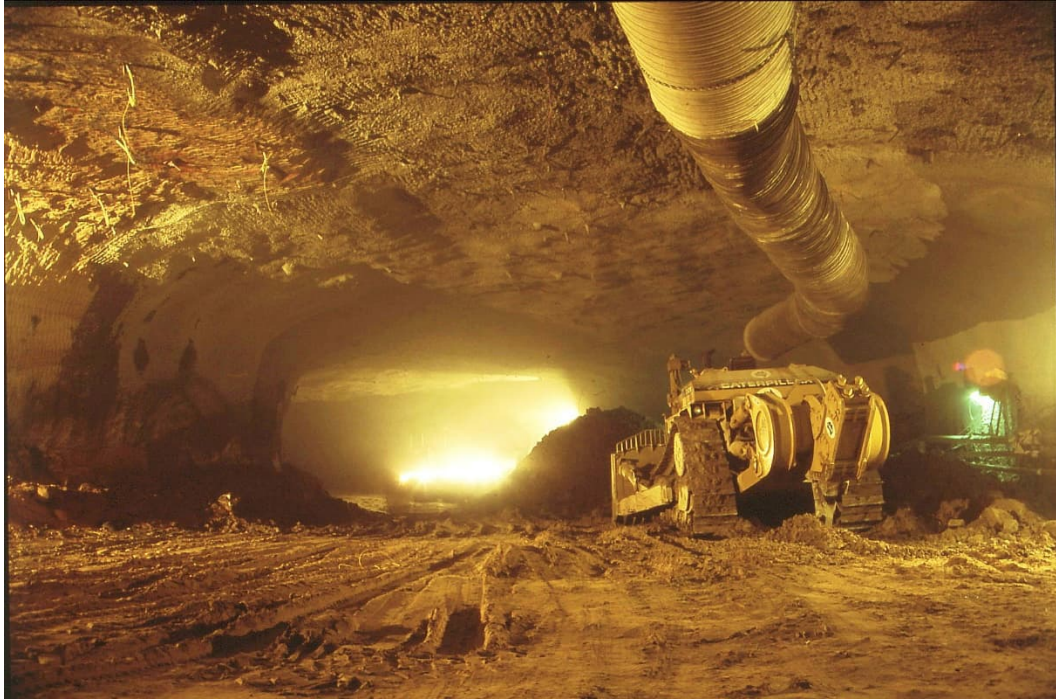
Figure 4: Commencement of bulk excavation of Hawkesbury Sandstone using impact ripping
