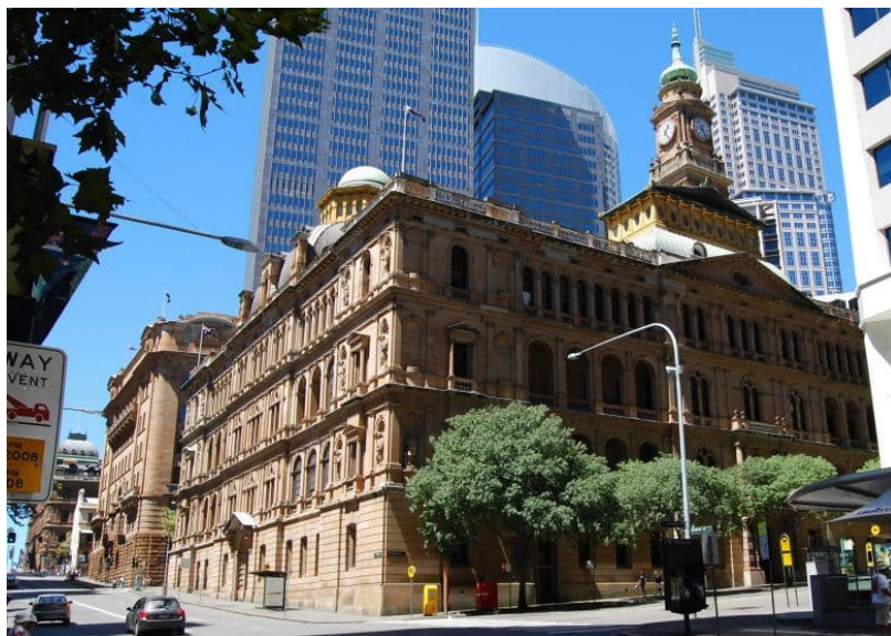
Figure 1: Photograph of existing heritage sandstone buildings being redeveloped
