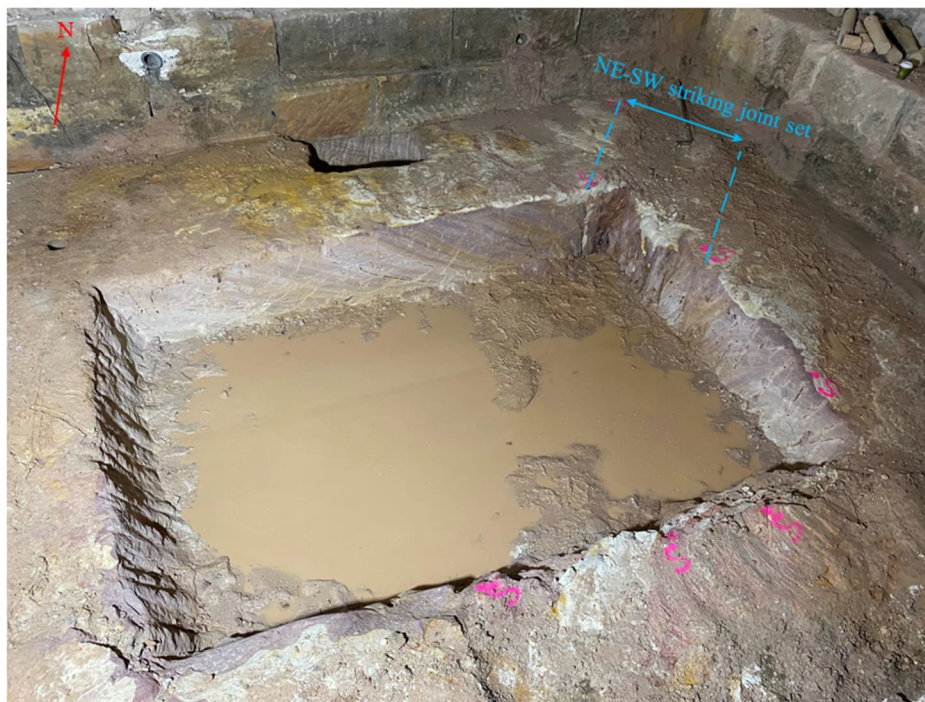
Figure 6: Typical jointing observed in trial trenches, refer to the blue hatched zone in Figure 7
