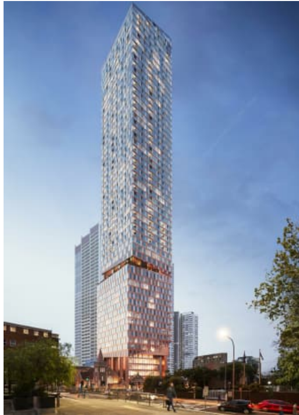
Figure 1: Rendered image of the proposed 59 storey tower (image courtesy of Woods Bagot)
