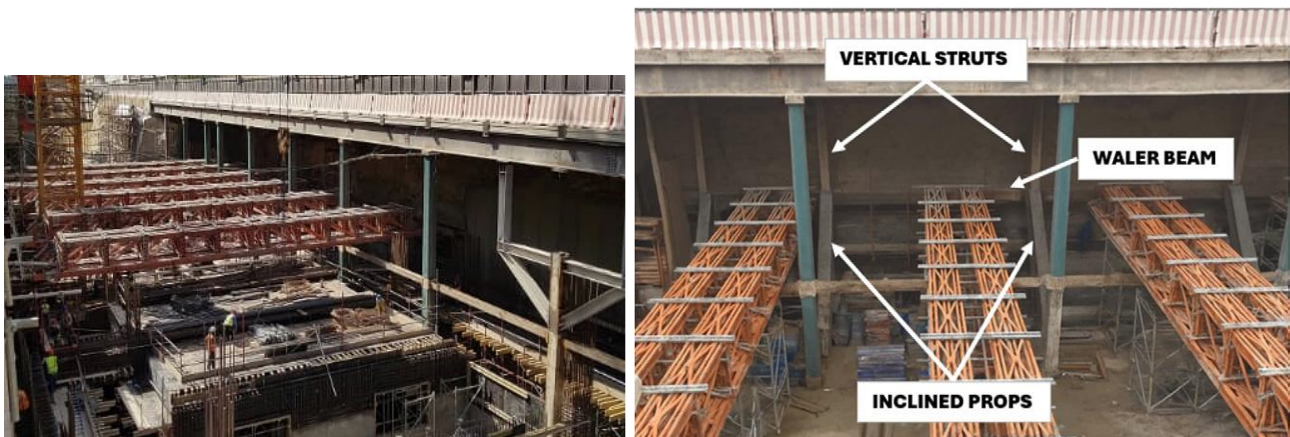
Figure 17: Excavation and retaining system during trial force reduction
