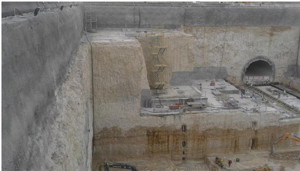
Figure 5: Another station excavation (30 m depth) in similar rock type (Breccia Limestone) and quality
