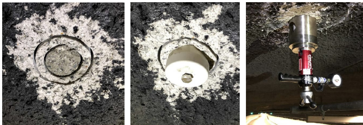
Figure A1: In situ testing of bond strength using a) drilled concentric core holes, b) mounting of a glued dolly to the end of a partially drilled core, and c) pull-testing, similar to the SS137243 test method.
