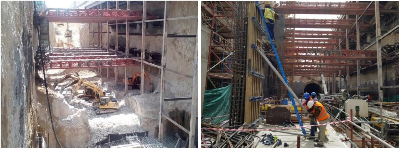
Figure 4: Left – Excavation about 2m above excavation bottom; Right – base slab already casted
