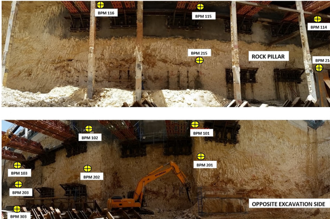
Figure 15: Monitoring prisms – rock pillar (top) and excavation opposite side (bottom) (upper props installed; brackets for support of lower props being installed)
