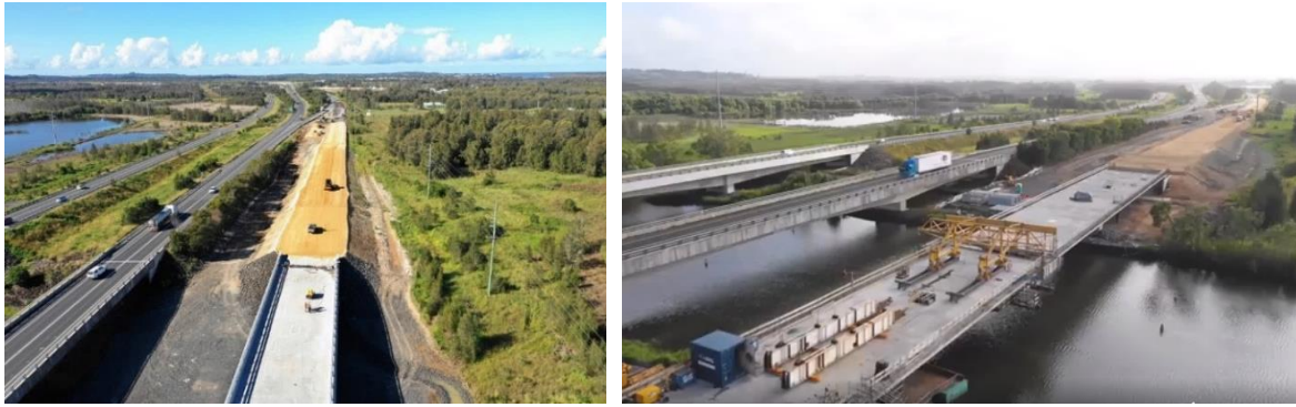
Figure 1: Southbound carriageway embankment and bridge construction at the second creek crossing
