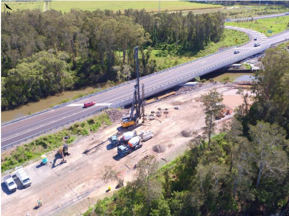
Figure 3: Concrete injected column (CIC) installation at the first creek crossing
