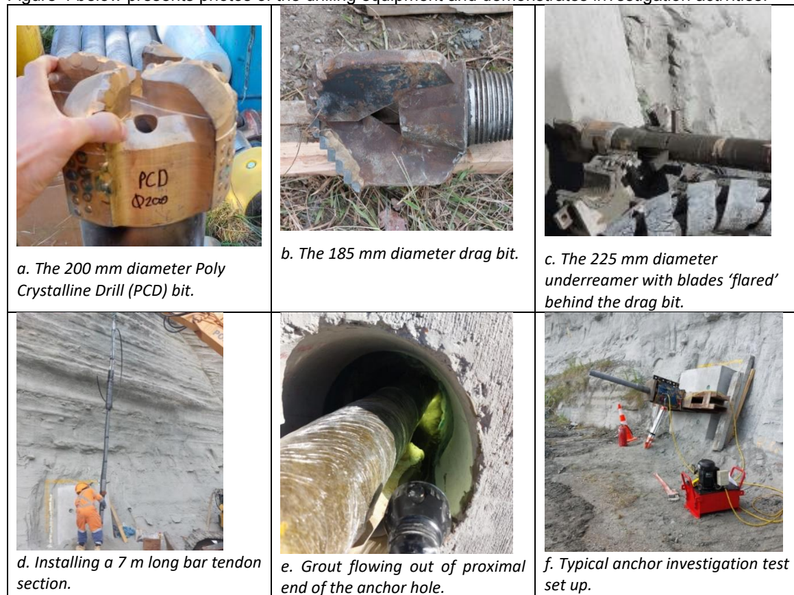
Figure 4: Construction and testing photos from investigation trial.
