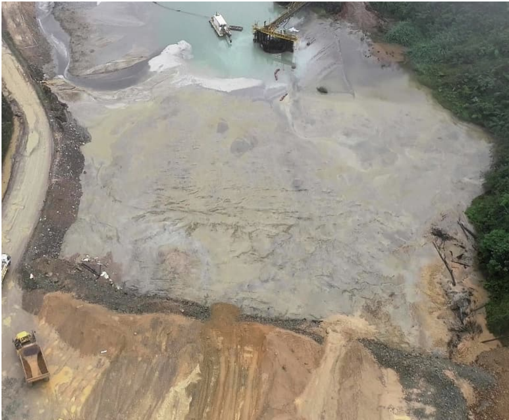
Figure 15: Mud-waving in progress
