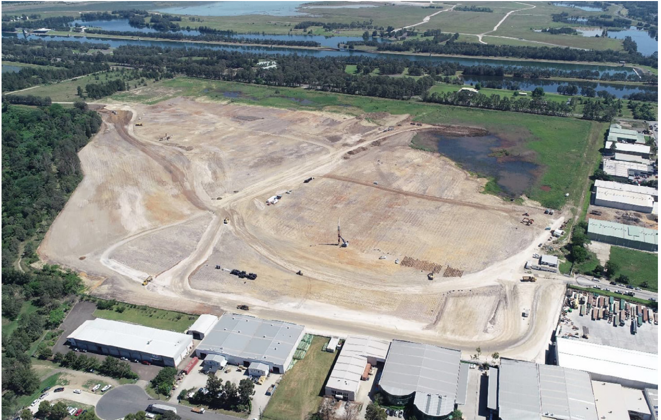
Figure 5: Aerial image at the start of the ground improvement works
