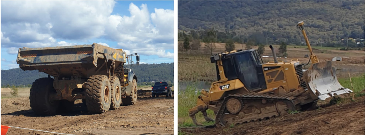
Figure 10: Earthworks moving equipment used initially
