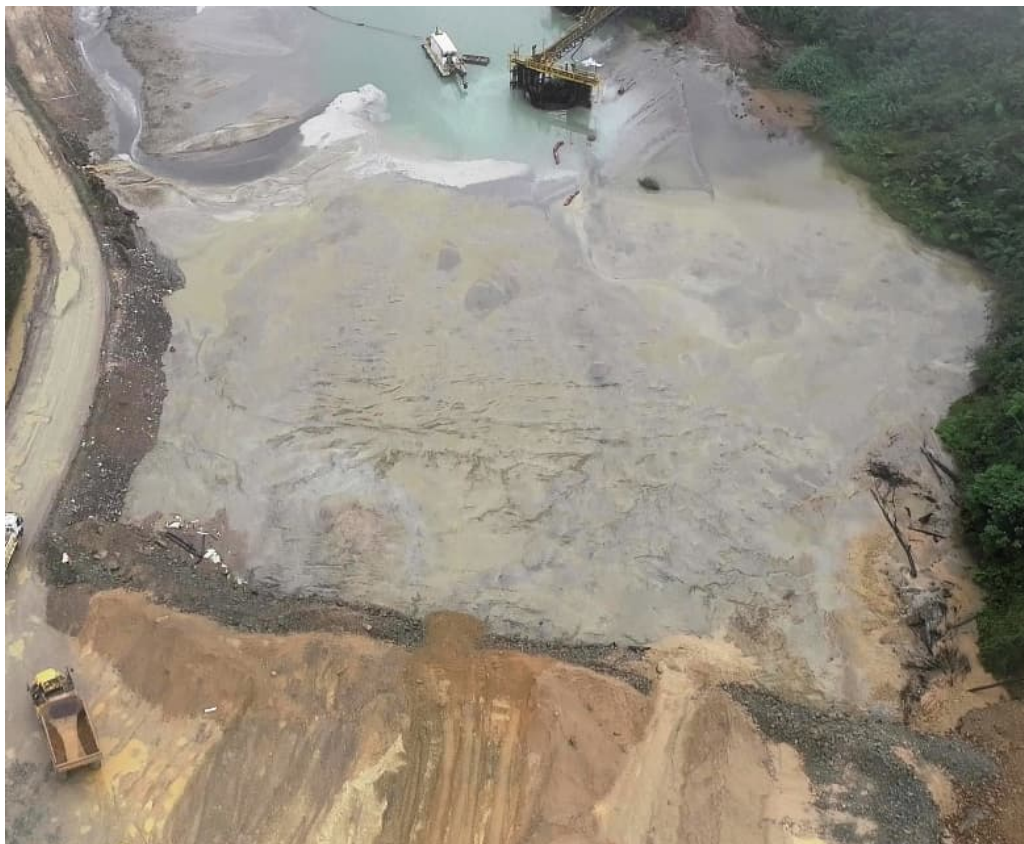
Figure 15: Mud-waving in progress
