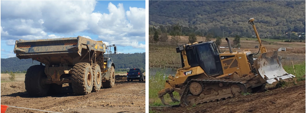
Figure 10: Earthworks moving equipment used initially
