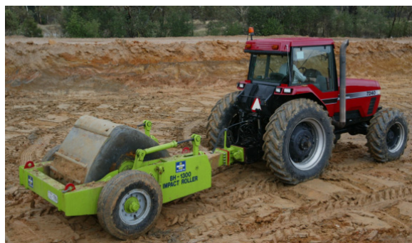
Figure 1. The 4-sided 'impact roller' towed behind a tractor
