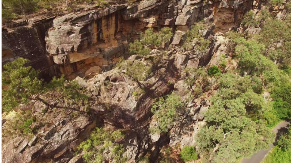
Figure 4. UAV photo showing cliffs and loose talus 40m above road (road lower right).
