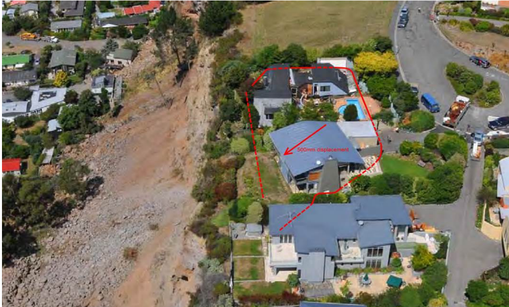
Figure 1. Low angle slip in loess affecting 3 houses in a cliff-top seismic amplification zone. Slip has displaced 500 mm horizontally with only minor vertical displacement despite having a back-calculated sliding FOS = 3. Most distant house has collapsed; central house has rafted en masse with shear passing underneath. Seismic amplification factor for this slide (from back-calculation) comes to over 1.6.
