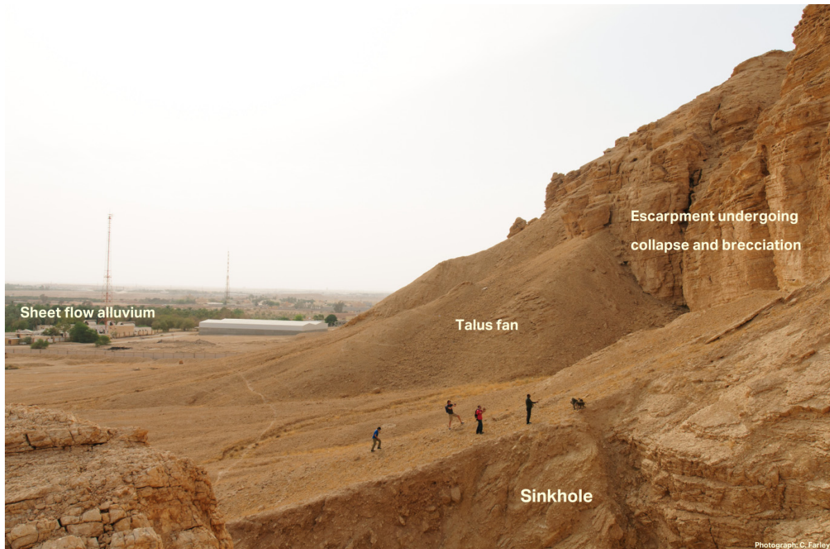
Figure 2. Escarpment showing large scale collapse of bedded limestone. Sinkholes were encountered at the foot of this escarpment in several locations.
