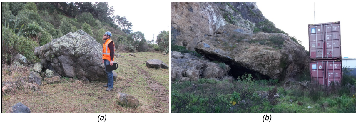
Figure 2. (a) This boulder is approximately 3 m 3 and is the result of rockfall from the continuous bluffs at the southern end of Wakefield Avenue; (b) This boulder fell as a result of the cliff collapse at the northern end of Wakefield Avenue. The boulder has landed at the base of the cliff immediately below where it was located; it has not rolled out towards Wakefield Avenue.
