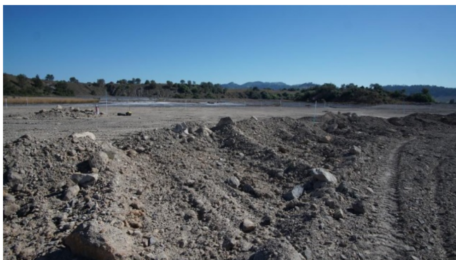
Figure 5. Capping works progress - secondary 1.0 m capping layer (August 2016)
