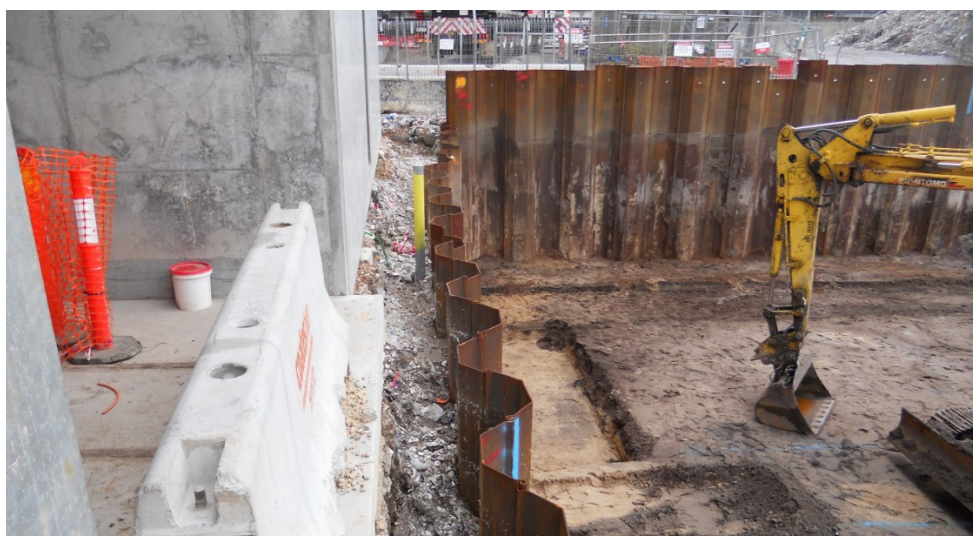
Figure 1. Rejects sump pit construction
