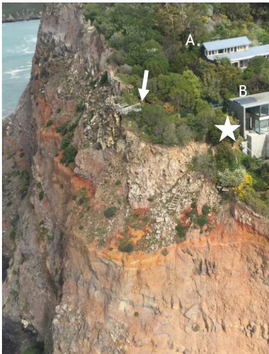
Figure 3(a). 65 – 85 m high sea cliff below Property A and B Whitewash Head, Scarborough. Note: timber framed lookout (24/09/2016 Aurecon).
