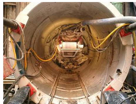
Fig 4. Segmental Tunnel Lining
