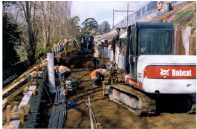
Figure 2 – Embankment Retaining Wall
