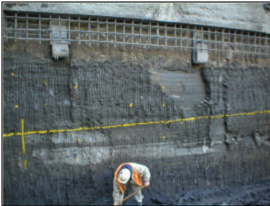
Figure 5– Typical exposed joint
