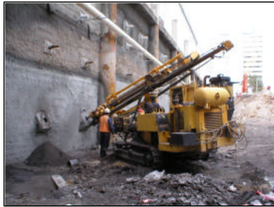
Figure 6– Drilling of the anchor holes
