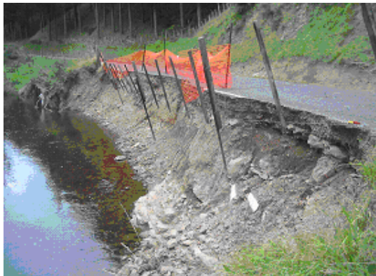
Photograph 1 Slip below road caused by undercutting of stream bank.
