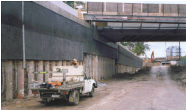
Figure 1 – Cut Retaining Wall
