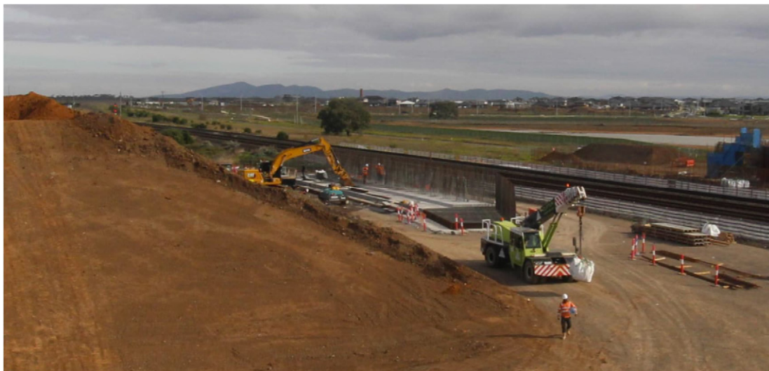
Figure 7: Casting of concrete base slab for south L-Shape wall (photo taken in June 2024)
