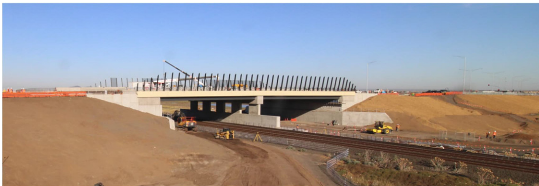
Figure 6: Ison Road flyover with completion of L-Shape walls, RSS walls and abutment backfilling (photo taken in February 2025)
