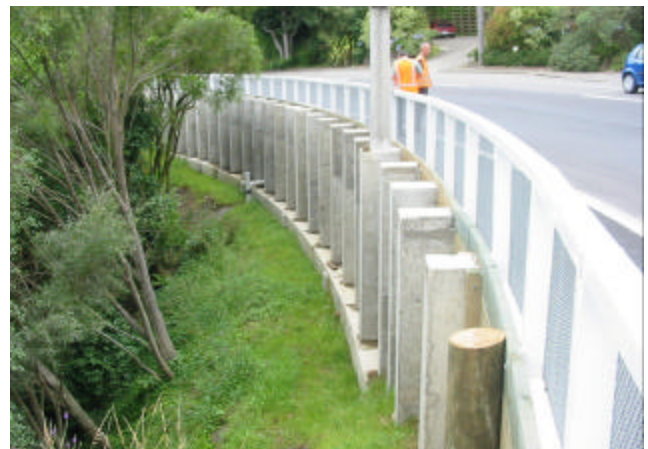
Figure 1. Completed Tied-Back Concrete Palisade Retaining Wall.
