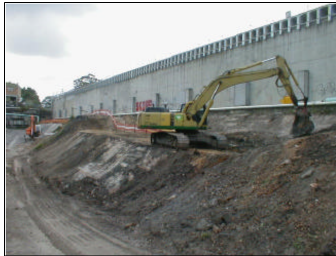
Figure 2 – RES and rail embankment prior to excavation
