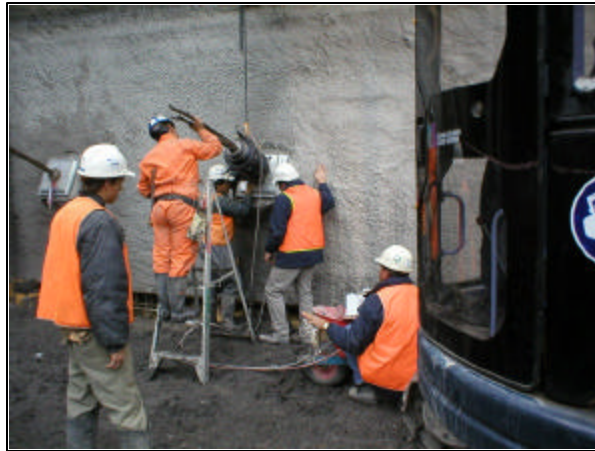
Figure 7 – Stressing of Anchor
