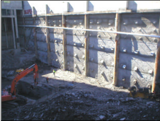
Figure 8 – Completed Permanent Multi-Anchored Retaining Wall
