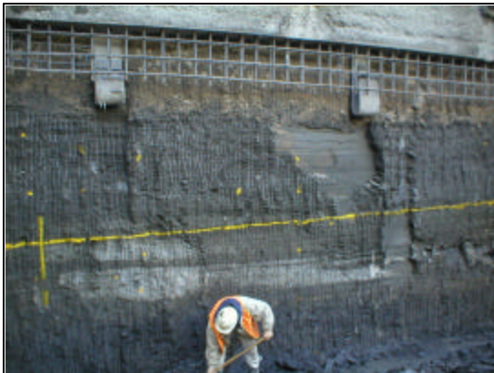
Figure 5 – Typical exposed joint
