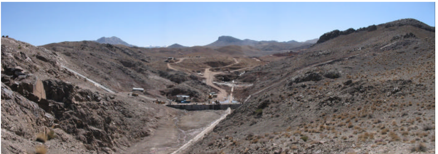
Figure 5 – Water retaining embankment (under construction) March 2004.
