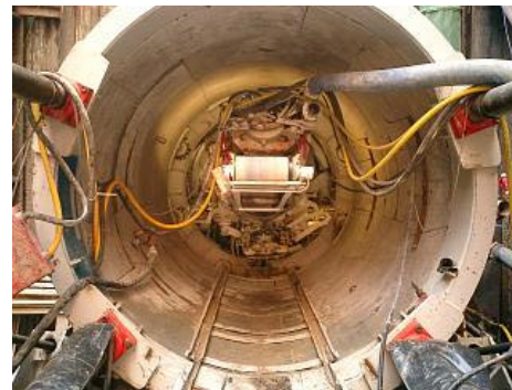
Fig 4. Segmental Tunnel Lining
