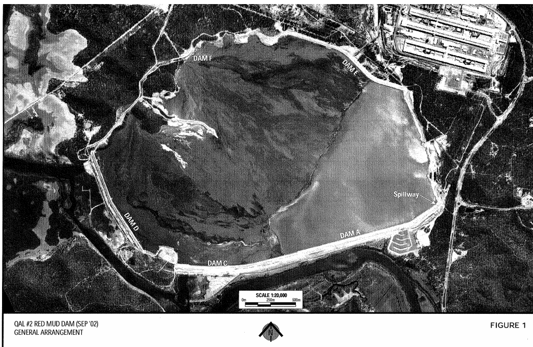
Figure 1 – QAL Red Mud Dam Number 2
