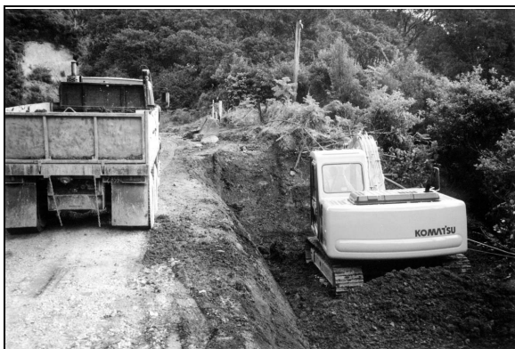
Photo 3. One lane remained open during construction.
