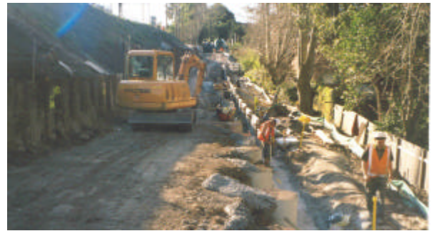
Figure 7 – Proposed base of RE block (left), and base of RE facing panels in front of piles (right)
