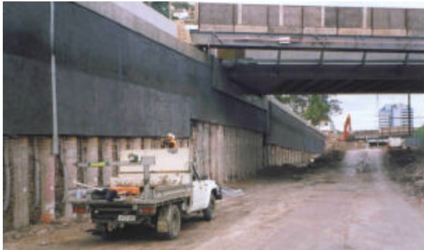
Figure 1 – Cut Retaining Wall
