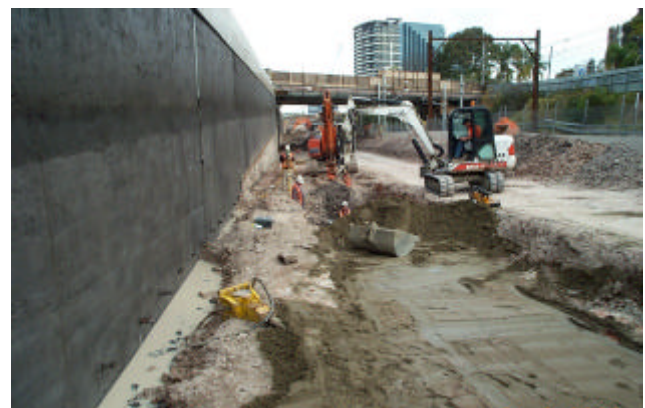
Figure 4 – Drainage Trench in front of Cut Wall
