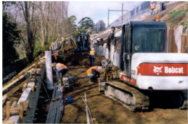
Figure 2 – Embankment Retaining Wall
