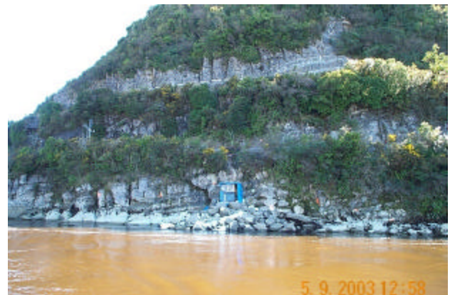
PHOTOGRAPH 1 - NORTH ABUTMENT LOCATION
