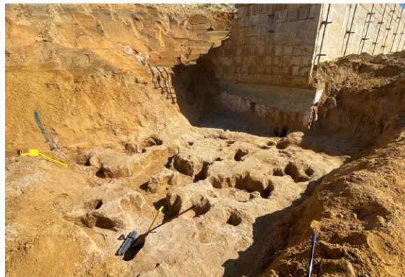
Figure 8: Example of a karstic features: (a) left: interior of Crystal Cave (Morey, 2025), a solution cave located 4 km from Pipidinny Road Bridge and (b) right: karstic features encountered during earthworks along YRE
