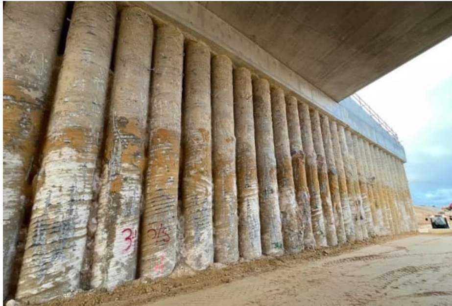
Figure 12: Contiguous Piles exposed after bulk excavation during construction of Pipidinny Road Bridge
