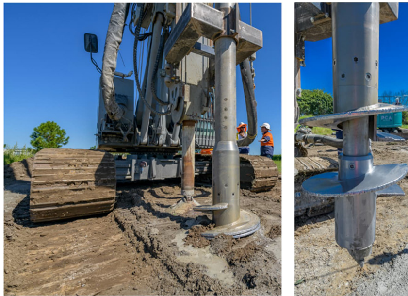
Figure 3: PAILE tool fitted to piling rig Comacchio CH450 with helical plates closed (left) and open (right).
