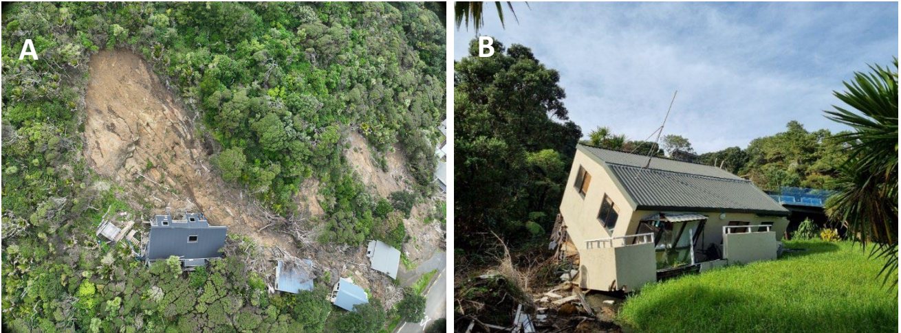
Figure 6: (A) Dwellings which have been rafted downslope from their original locations remaining relatively intact. (B) Photograph of a dwelling which has been rafted and toppled over by a landslide, with lower-level of the dwelling completely destroyed, while the upper-level remains mostly intact.
