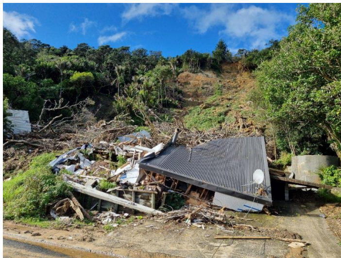
Figure 1: Complete destruction of a dwelling in Muriwai resulting from debris flow impact.
