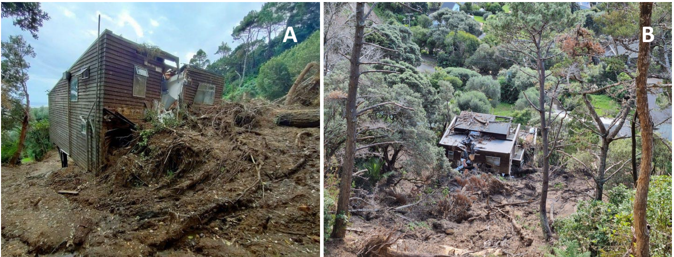
Figure 7: Photographs of a dwelling which has been impaled by a tall pine tree. Both photos are of the same dwelling taken at ground level and from the headscarp, respectively.
