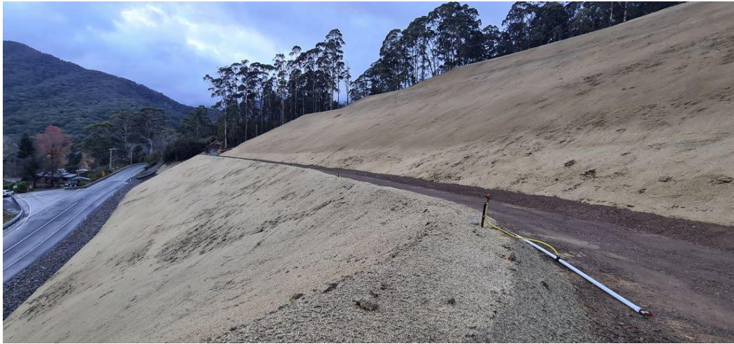
Figure 9: Far field view of remediated slope (bench 10 m wide)
