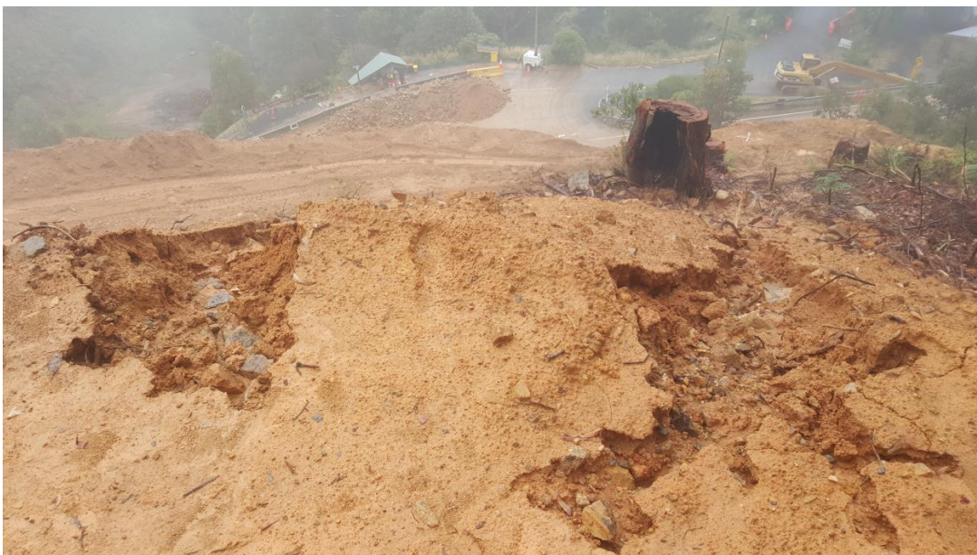
Figure 8: Gully erosion after heavy rain, 18 January 2023
