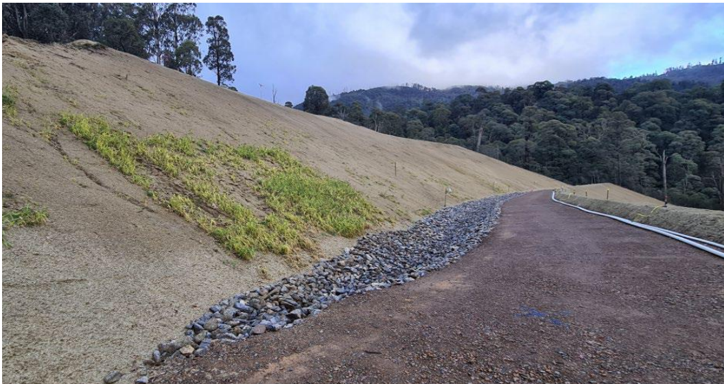
Figure 10: View along completed bench (bench 10 m wide)
