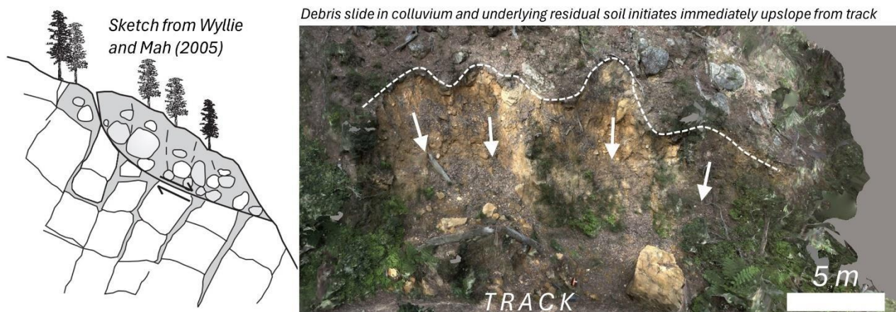
Figure 5: Conceptual sketch and example of a debris slide in colluvium and residual soil
