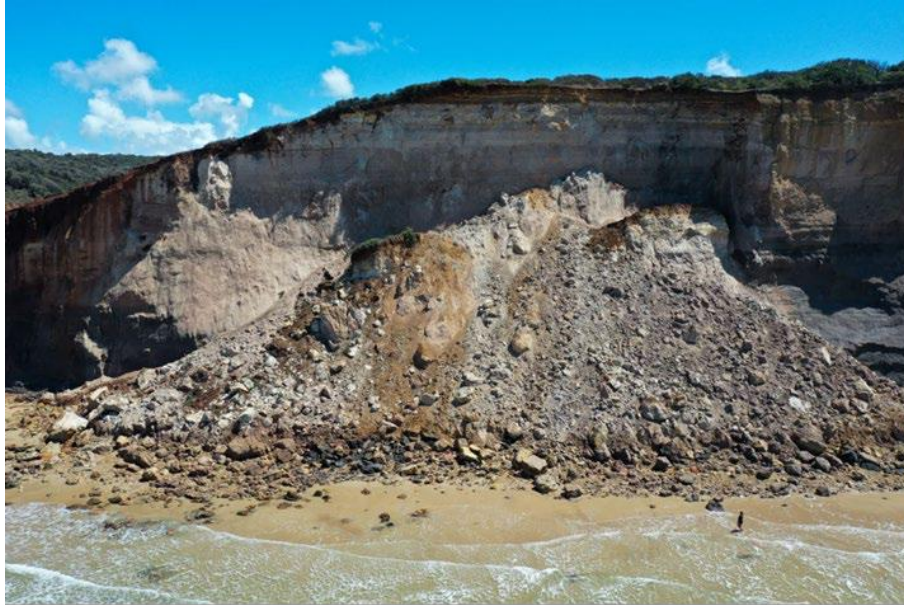
Figure 2: A very large coastal cliff collapse / rockslide of approximately 40,000 m 3 occurred at Jarosite Headland in Victoria. Only 100 m to the southwest of the site of a fatal rockfall of only 2 m 3 occurred killing 1 person and injuring 2 others just a month earlier.
