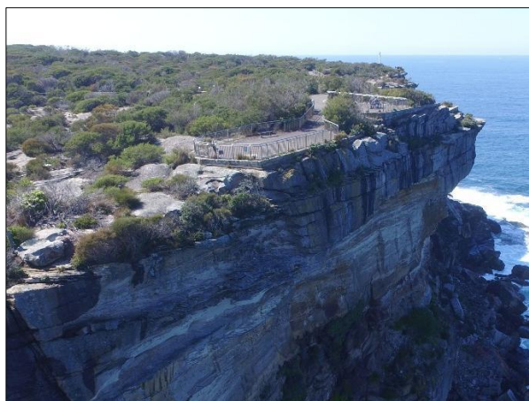
Figure 6a Lookout One pre construction (looking east, image courtesy of NPWS, 2016)
