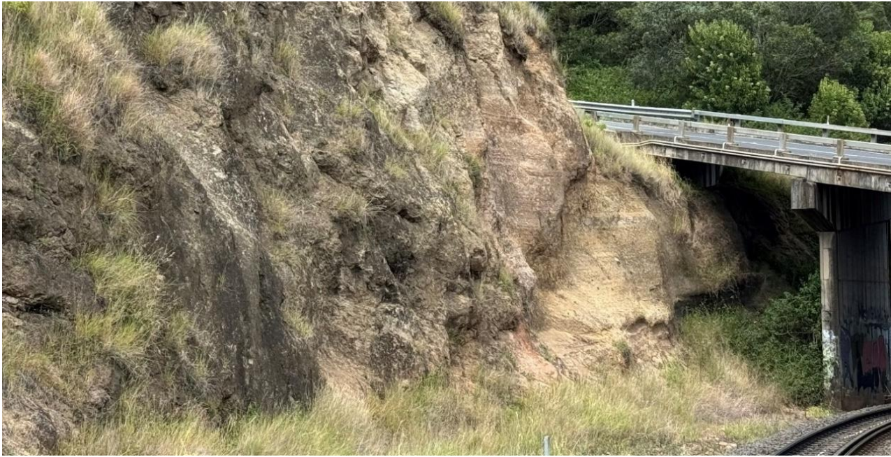
Figure 4: Typical rail cutting in Tuff
