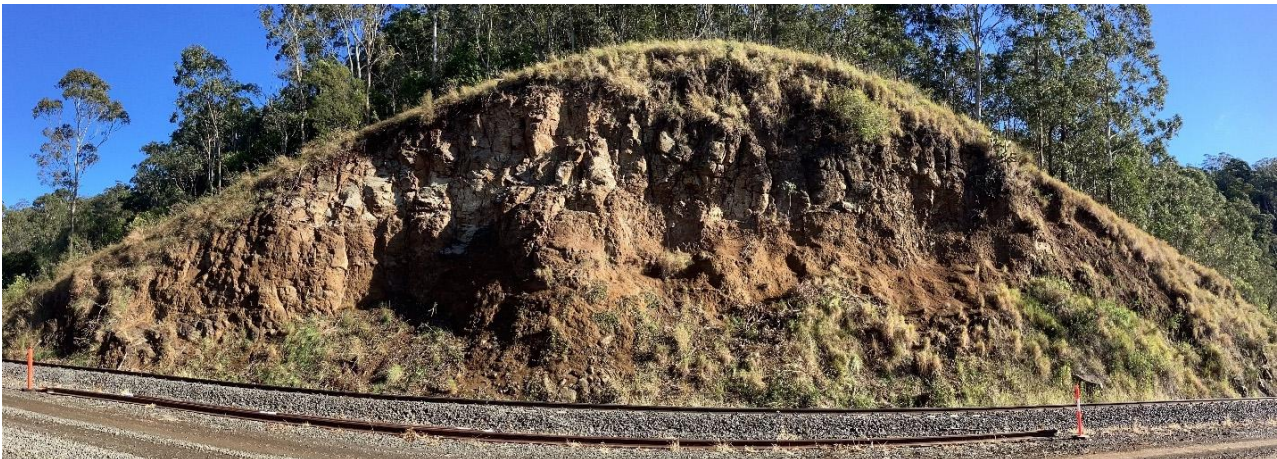
Figure 3: Rail cutting showing competent basaltic blocks progressively undercut
