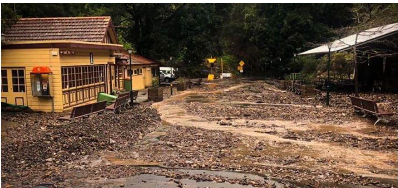
Figure 2: Flooding at Jenolan Caves in February 2020 looking towards the western side of the Grand Arch
