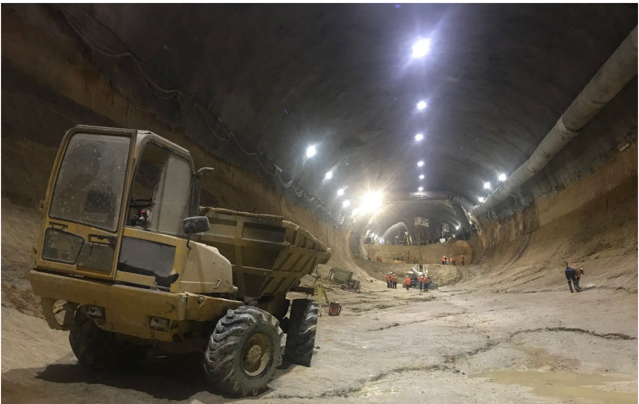
Figure 11: View of the final excavation profile of the Barangaroo crossover cavern.
