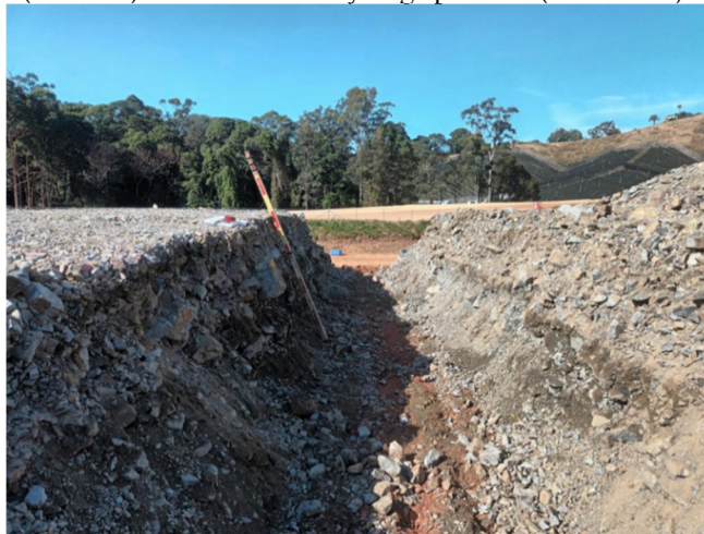
Photograph 6 - Trial 1 test pit showing good trench side definition
