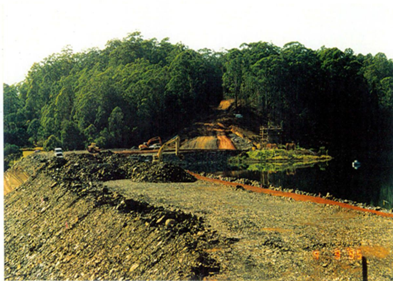
Photograph 2 Unprocessed rockfill dam embankment under construction at Karangi circa 1995
