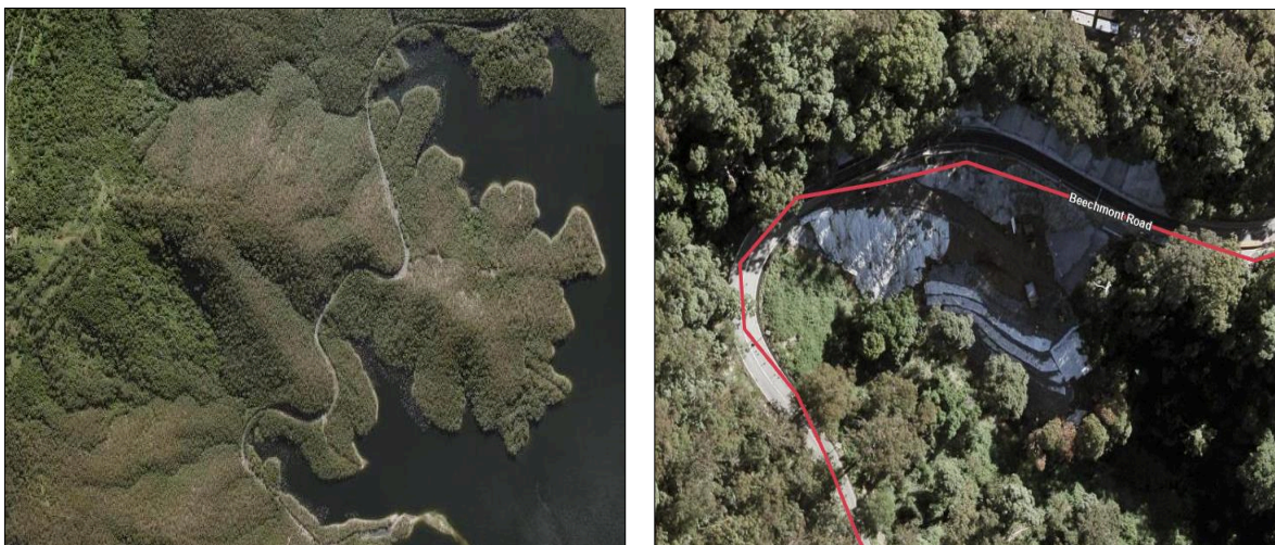
Figure 4: Images of required project data Left - state imagery / Right - road control line.
