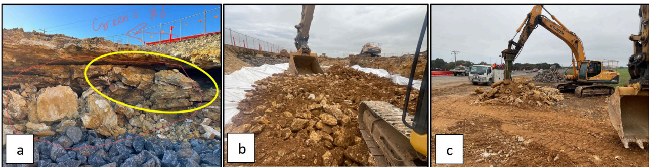
Figure 4: Failing aeolianite blocks (a), Aeolianite and caprock used as the 'plug' backfill (b) and (c)
