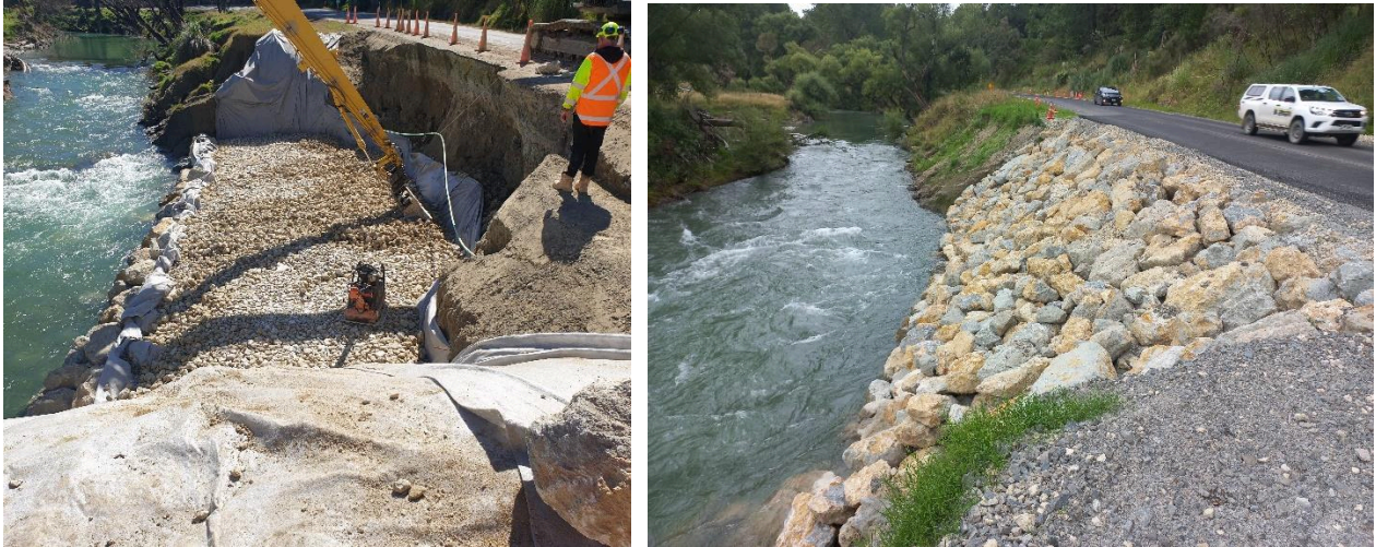
Figure 7: Waikaretaheke Stream construction photo (left) and completed photo (right)
