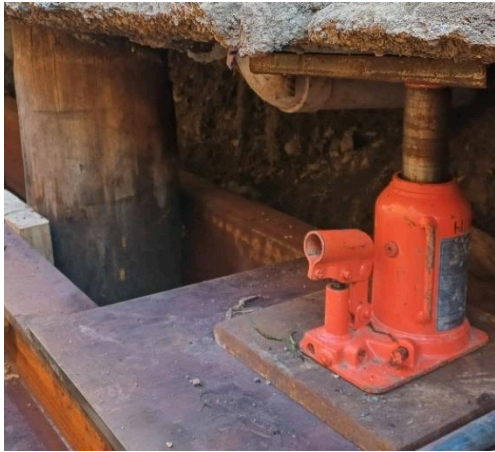
Figure 4: (a) Jacks between jacking beam and underside of the rib-raft foundation and (b) Pile Cut
