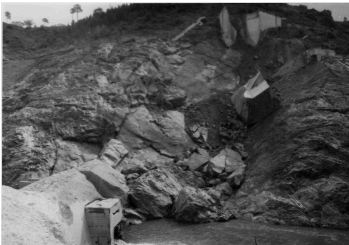
Figure 2: Malpasset Dam remains of the left abutment (Mary, 1968)
