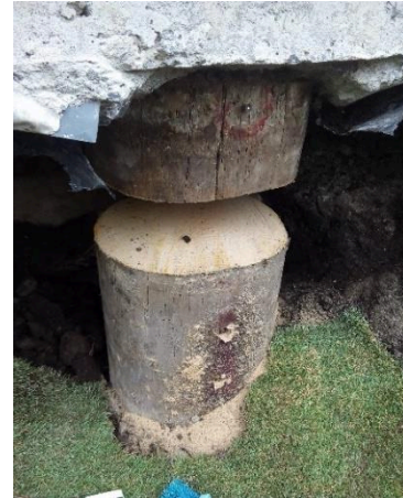
Figure 4: (a) Jacks between jacking beam and underside of the rib-raft foundation and (b) Pile Cut
