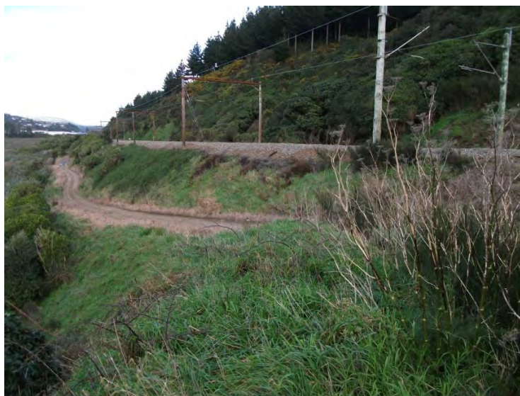
Figure 1: Existing high risk rail embankment
