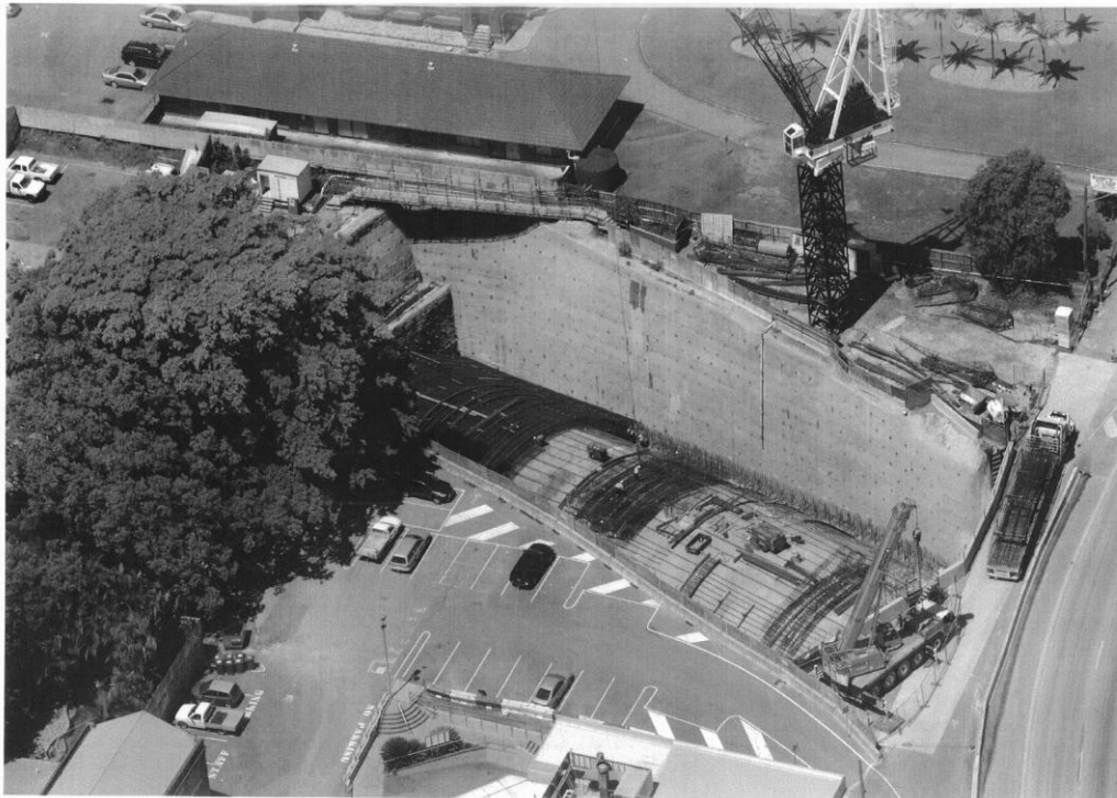
Figure 3: Site constraints shown in an aerial photograph taken during construction of the capping slab. Note the mobile crane, tower crane and church hall.
