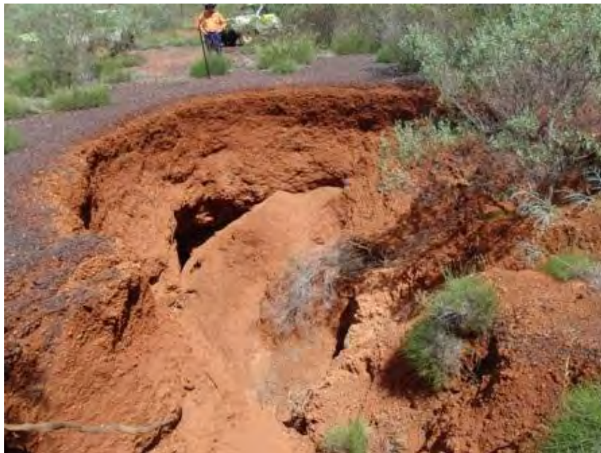
Figure 2: Active drop-out sinkhole located some 15km from the proposed plant site.
