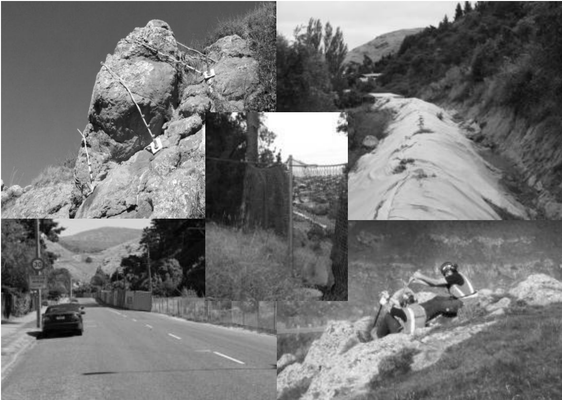
Figure 4, typical emergency protection measures carried out. (center) temporary catch fence, (clockwise from top left) rock anchor and cable tie back, temporary earth bund, rock scaling, and shipping containers as a temporary protection barrier (Leon Gerrard)
