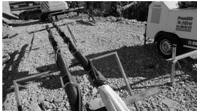
Figure 4: Filter Sock Wrapped On Soil Nail Sheathing for Figtree West
