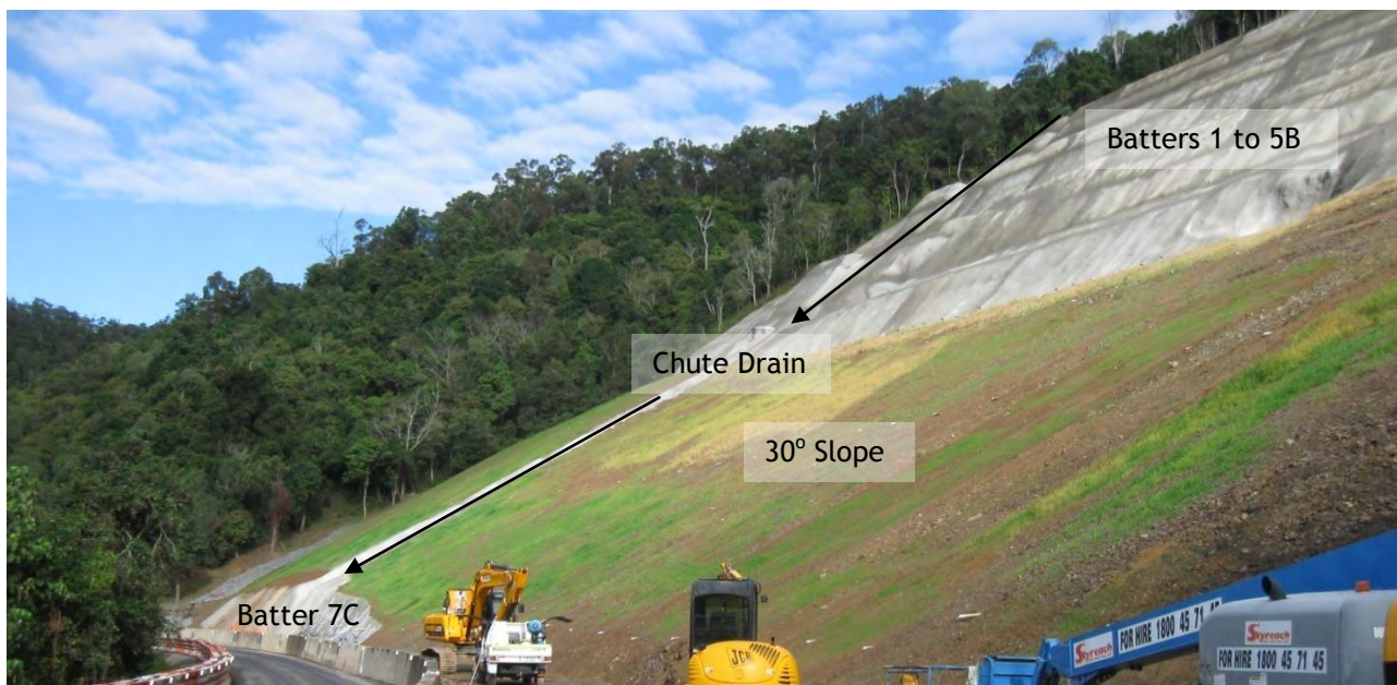
Photograph 1: General Site Appearance Looking South
