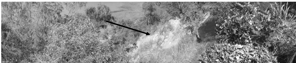
Figure 1: A view of the landslide from the top of the bluff.
