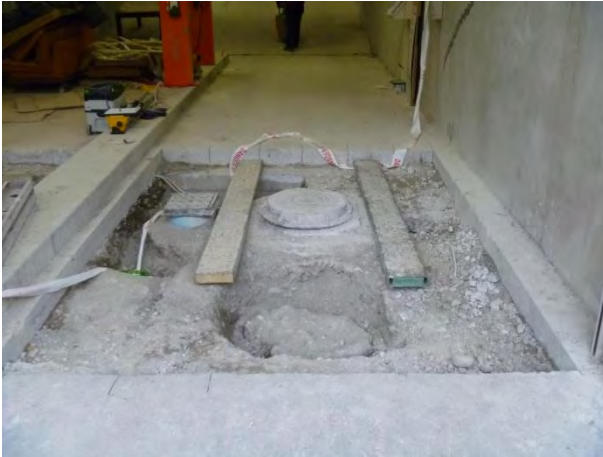
Figure 2. Exposed pile
