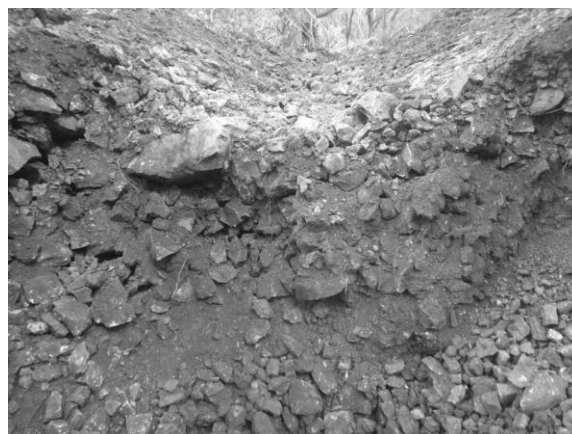
Figure 3: Loose Fill Materials at Base of Excavation in Figtree West
