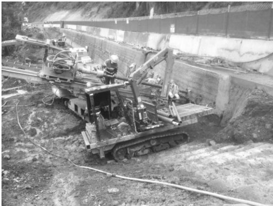
Figure 5 (left): Temporary Soil Nails at Cut 18; Figure 6 (right): Installation of Permanent Soil Nails at Cut 18 West Drilling rigs mounted to track excavators were specially designed to access normally unreachable soil nail locations, especially at Cut 18 West which required five (5) rows of soil nails below the highway (Figure 6).
