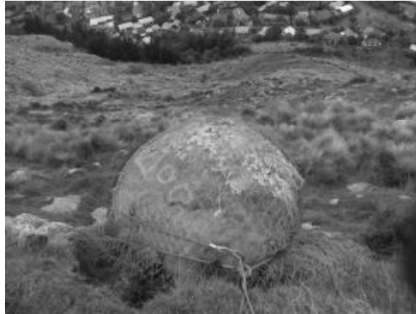
Figure 7, a large unstable boulder approximately 1.5m in diameter held in place by steel mesh and cables (Leon Gerrard)
