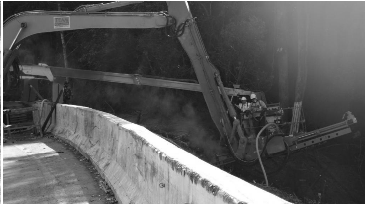
Figure 5 (left): Temporary Soil Nails at Cut 18; Figure 6 (right): Installation of Permanent Soil Nails at Cut 18 West Drilling rigs mounted to track excavators were specially designed to access normally unreachable soil nail locations, especially at Cut 18 West which required five (5) rows of soil nails below the highway (Figure 6).
