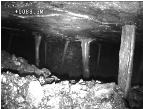
Figure 3a: Intact Workings
