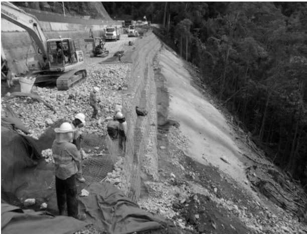
Figure 7 (left): Rockfill and TERRA® Mesh at Cut 18;
