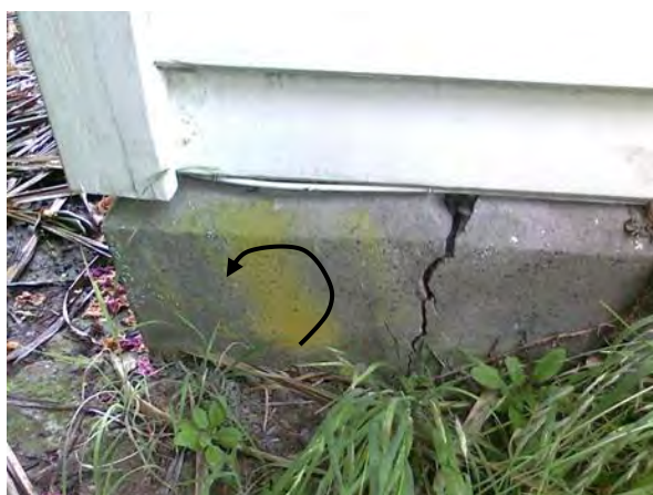
Figure 7: Rotating concrete ring beam foundation
