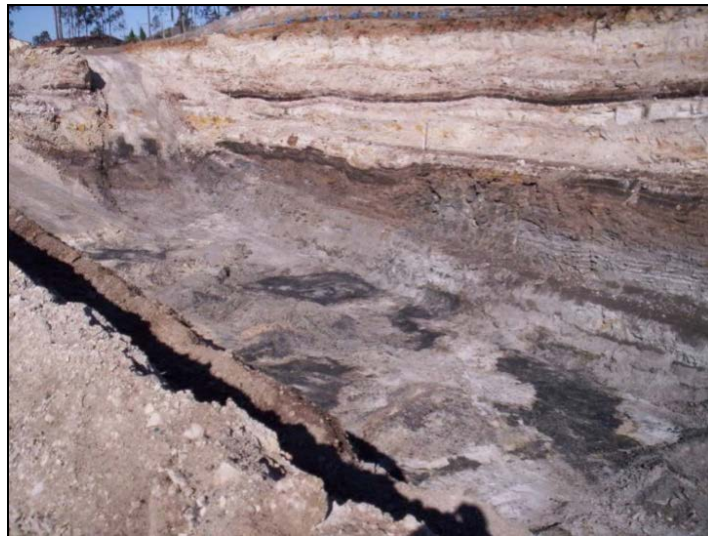
Figure 1: Earthworks remediation of shallow mining to the west of Newcastle. Note the undulations in upper seams in cut batters due to subsidence, and remnant coal pillars exposed in the floor of the excavation
