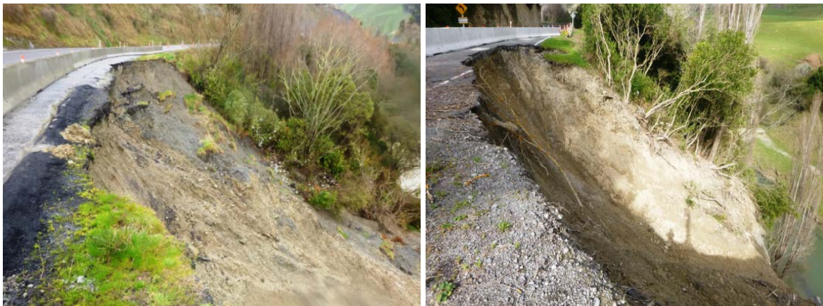
Figure 5: Observed damage at slip sites #14 (left) and #22 (right)
