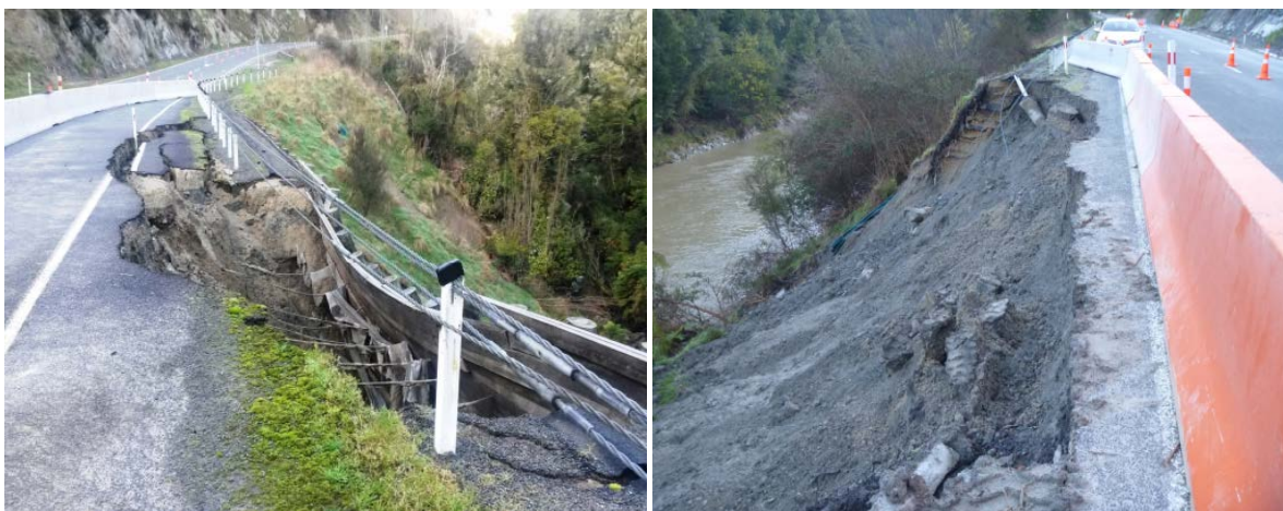
Figure 5: Observed damage at slip sites #14 (left) and #22 (right)
