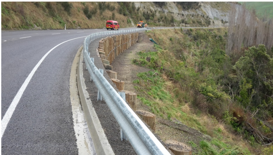
Figure 11: Photograph of completed remedial works at Site #14
