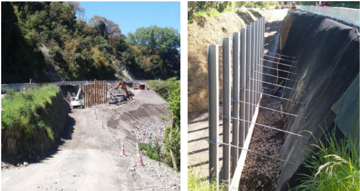
Figure 9: Photographs of Site #16 (left) and Site #22 (right) during construction
