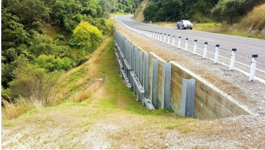
Figure 12: Photograph of completed remedial works at Site #24/25
