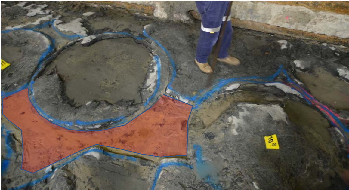
Figure 4: Example of top surface of base block (red indicates columns not overlapping)
