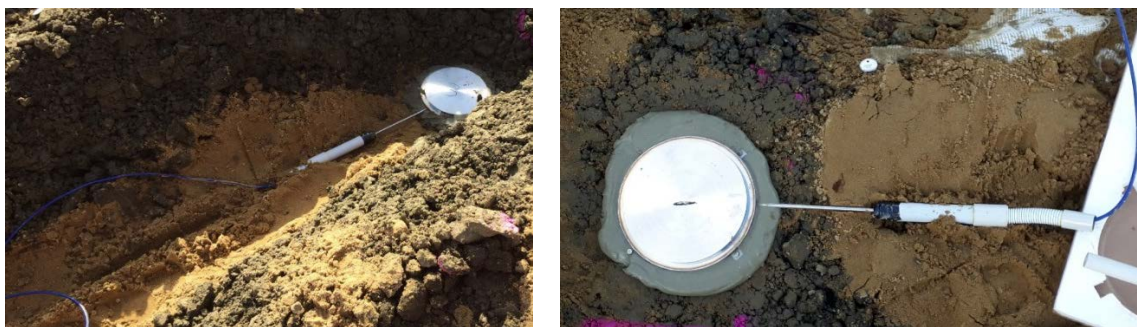
Figure 7: Pressure Cell Installation
