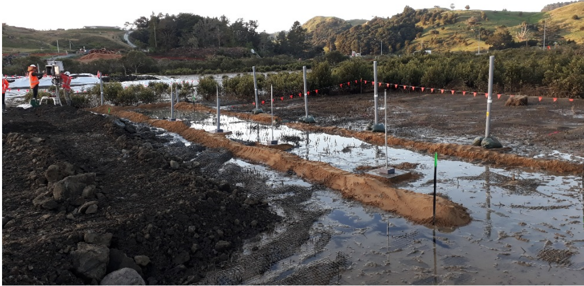
Figure 4: SAA and Settlement Plates Installed
