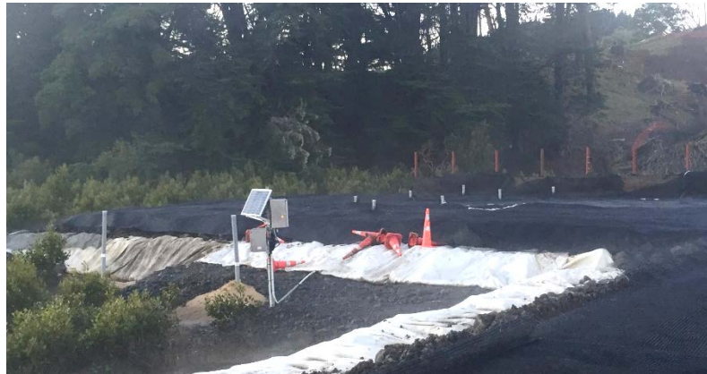
Figure 5: Settlement Plates at different stages
