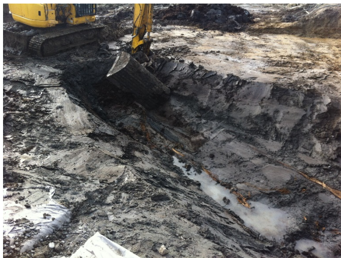
Figure 2: Excavation of peat, including intact logs.
