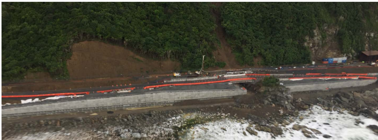
Figure 8: Aerial photograph of 80% complete NFC G-Wall site (photograph taken 10 April 2018)
