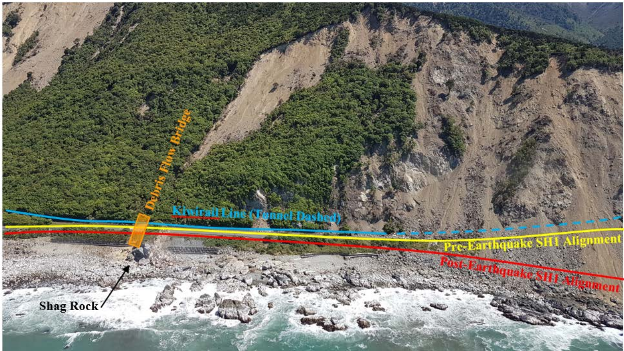
Figure 3: Photograph of area south of Ōhau Point (14 December 2016) showing earthquake related damage with approximate locations of pre-earthquake and post-earthquake road alignment
