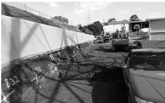
Figure 14. North Dynon lead soil nail wall
