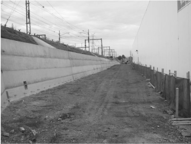
Photograph 1. Finished soil nail wall
