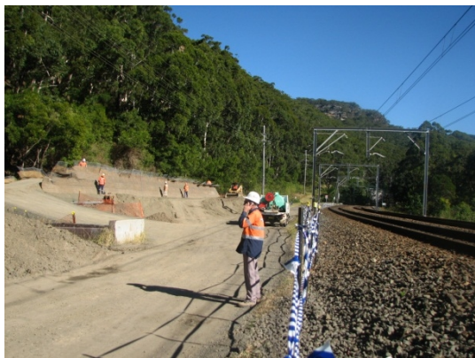
Figure 20. Embankment two: 50 meters long
