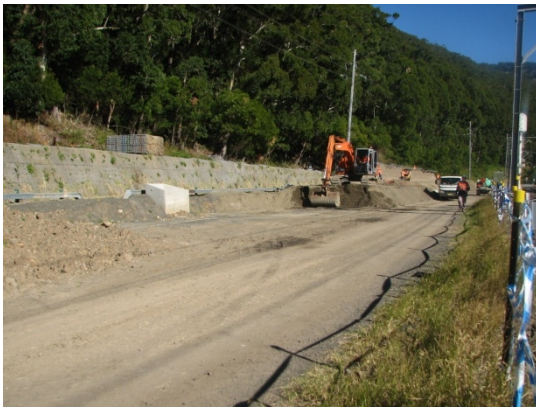
Figure 19. Embankment one: 65 meters long
