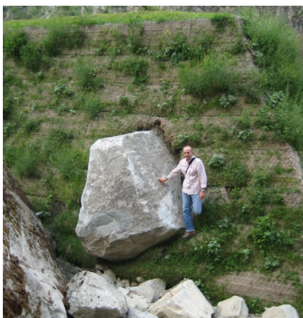
Figure 4. Close up of the block which struck the upstream embankment (7,500 kJ impact)
