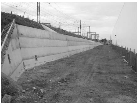
Figure 10. Maribyrnong viaduct soil nail wall
