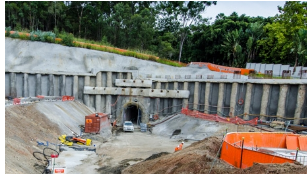
Figure 6. The temporary Conveyor Tunnel Portal with berm
