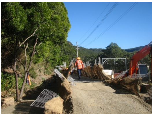
Figure 15. South access ramp to embankment
