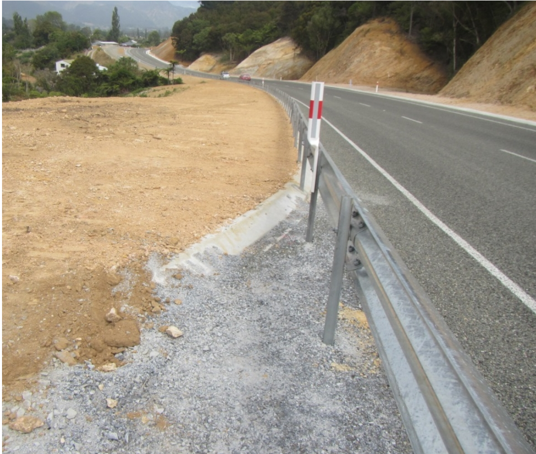
Figure 3. Birds Hill SH60 post-remediation construction, December 2013.
