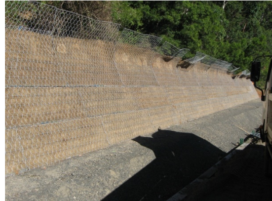
Figure 17. Factory fitted biodegradable facing layer which retains good quality topsoil
