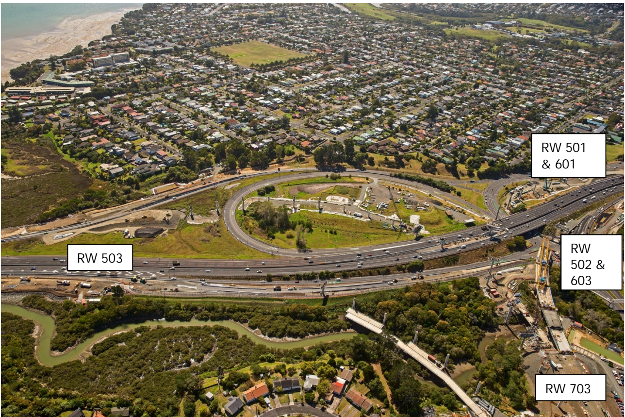
Figure 4. Aerial view of the Great North Road Interchange and northern retaining walls looking north.
