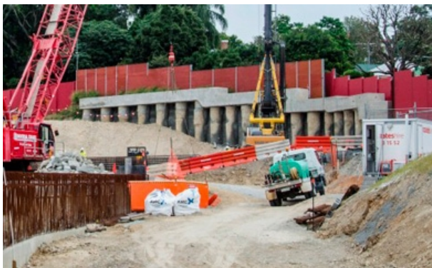
Figure 5. The Eastern Soldier Pile Wall with berm
