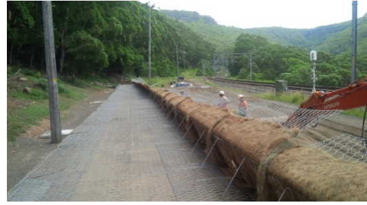
Figure 16. The mesh front face acts as framework during construction
