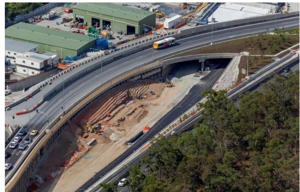
Figure 4. The Western Trough Structure with berm
