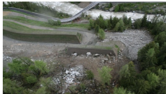
Figure 2. Aerial view of two embankments after the collapse of blocks (>10,000 kJ), Cogne, Italy
