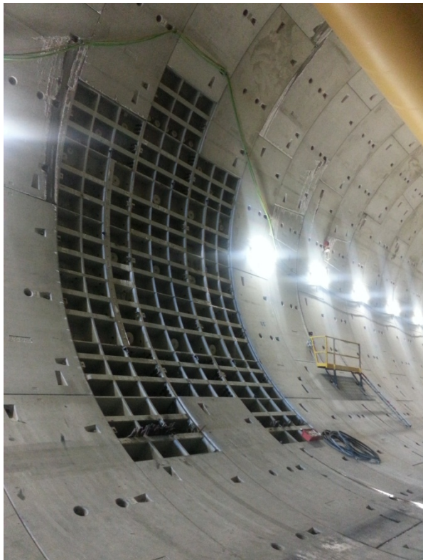
Figure 3. Temporary steel segments installed at cross passage opening.
