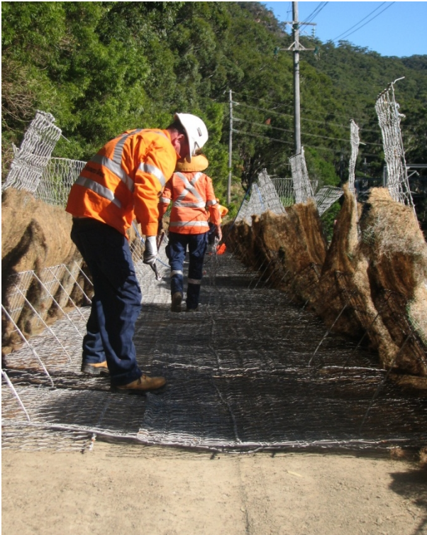
Figure 14. Assembly of Green Terramesh units
