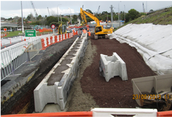
Figure 6 Stone Strong block placement for RW502.
