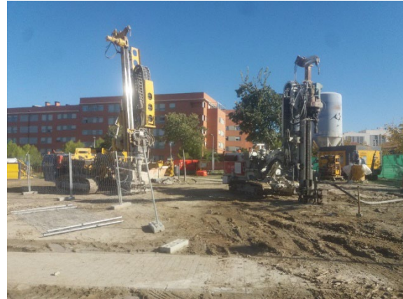
Figure 6. Test area for injections. Treatment type B.
