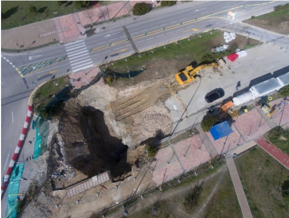
Figure 5. Start of the works. Treatment type A.
