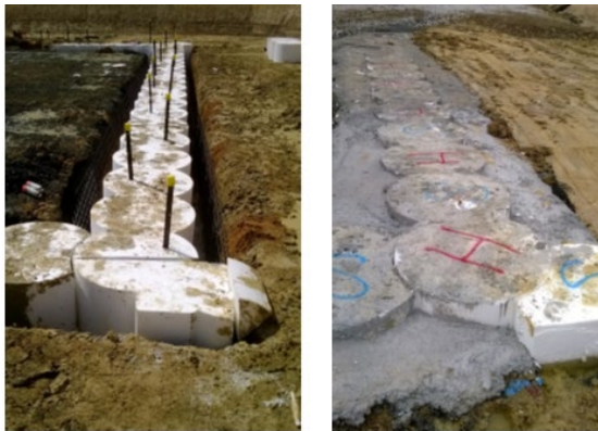
Figure 4b. Typical guidewall installation and construction
