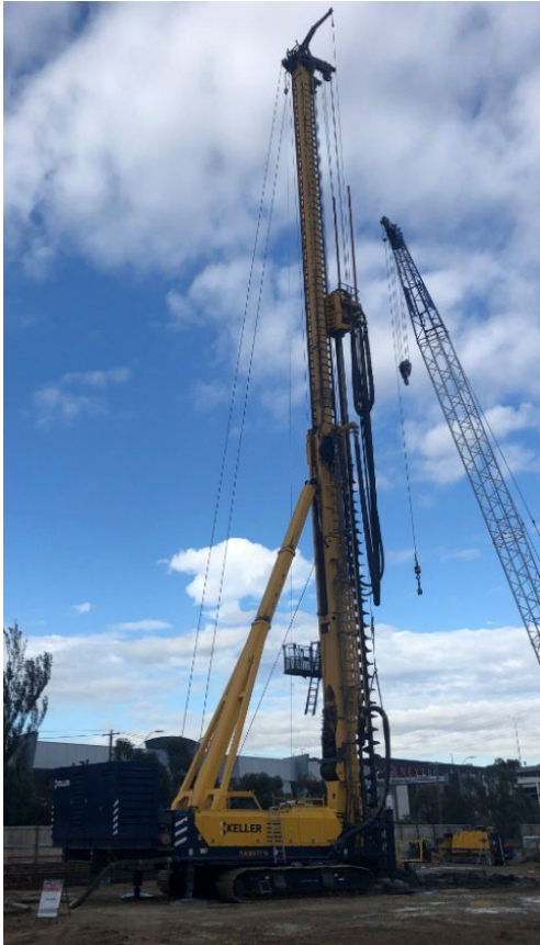
Figure 1. The Fundex F3500 piling rig
