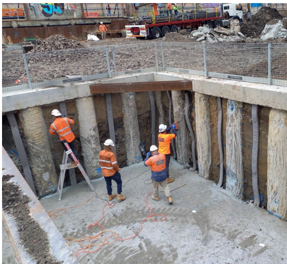
Figure 12. Core excavation
