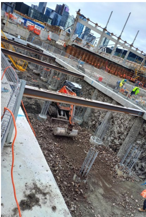
Figure 13. Core excavation
