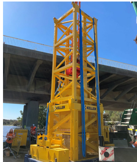
Figure 3. The 20T test hammer set up for dynamic load tests
