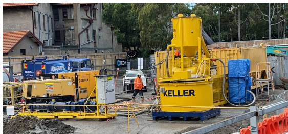
Figure 8. Mixing plant on site
