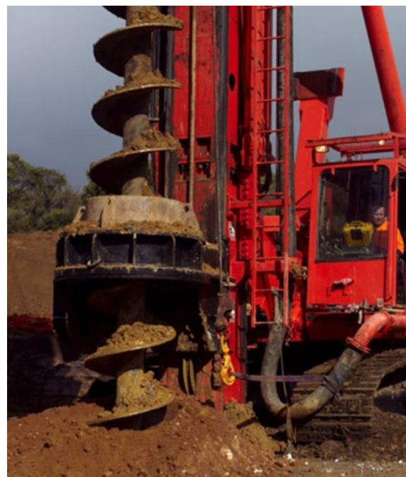
Figure 1. CFA pile drilling.
